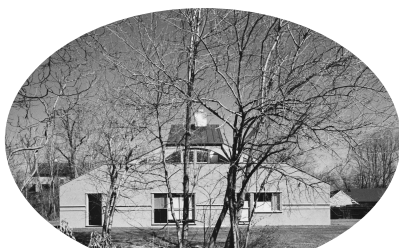
South elevation of Vanna Venturi House
