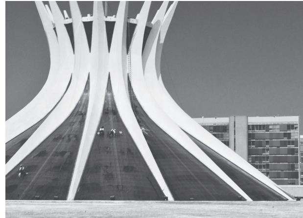
It has been half a century or more since these buildings were constructed with the authorial ambition of creating an 'island'. However, they are aging today, both physically in terms of their corroding structures and ideologically of the socio-cultural movement they once represented.
